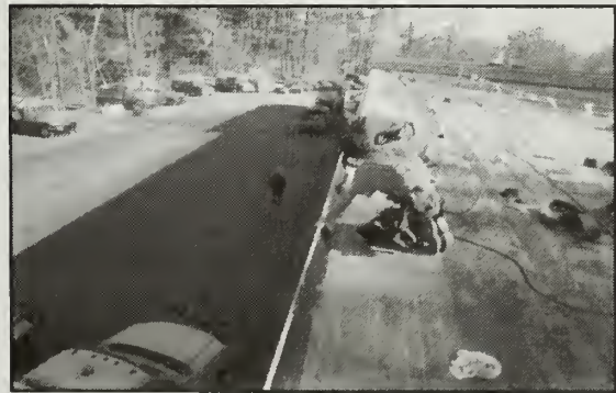
Below: (L) .040 aluminum edge was installed (R) Rubberized black granule modified bitumen cap sheet was installed over two base piles
